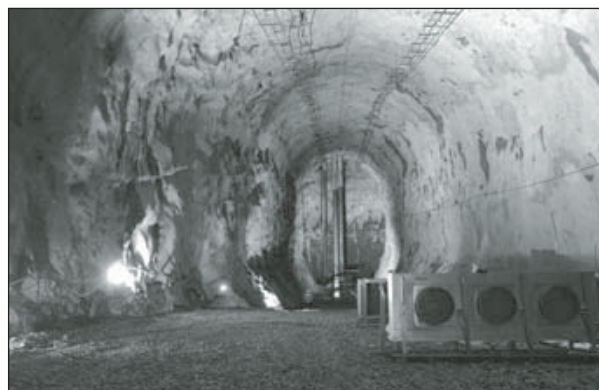
Figure 5. Cooling fans in the cavern
