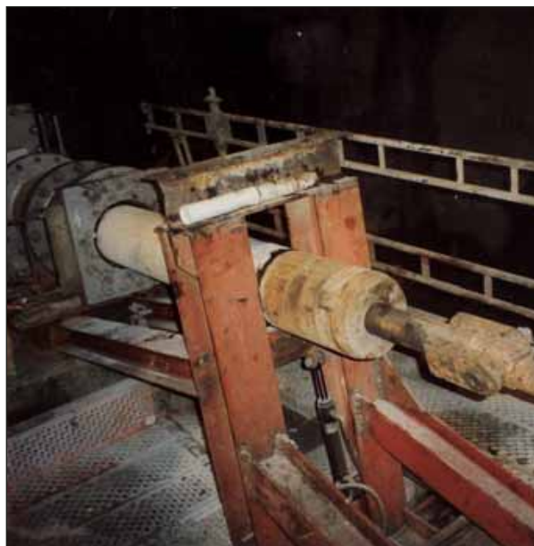
4. The drill string is being pulled through the seal tube system by the winch, prior to the reaming operation.
