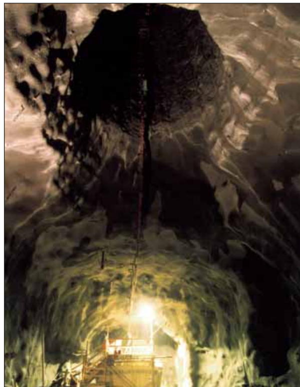
Piercing area - shaft excavation completed
