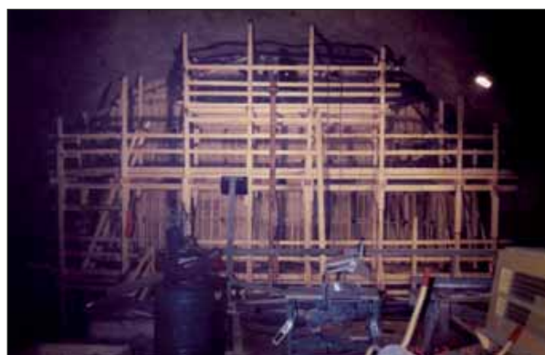
Concrete plug casting
