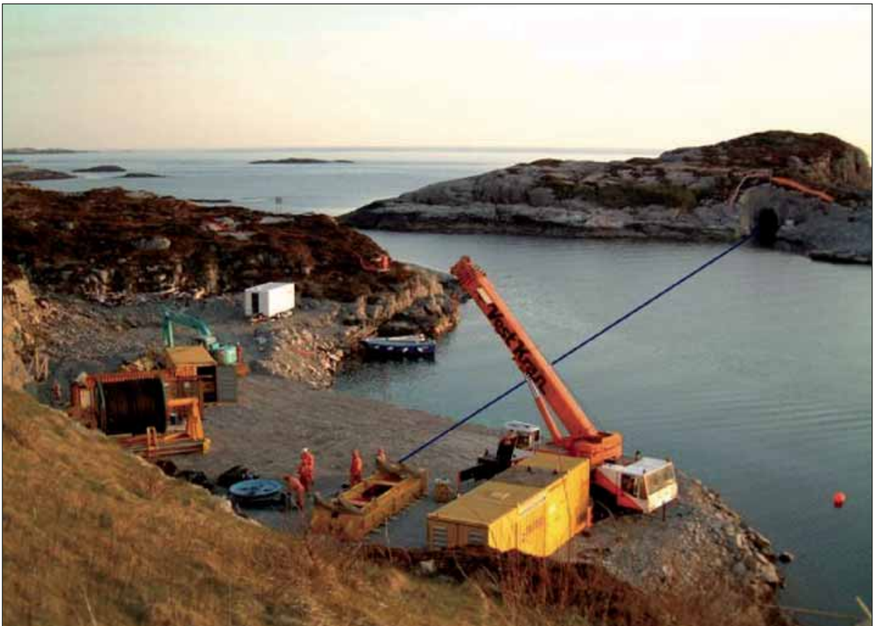
Figure 16: Overview picture from the Kollsnes landing site prior to the pipeline pull-in. Pull-in wire direction illustrated with dark line. (Photo: Statoil)
