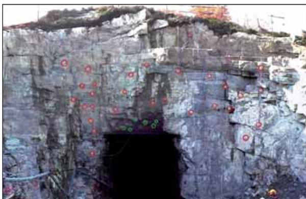
Figure 9: Installed rock support in the tunnel entrance open cut area. (Photo illustration: Norconsult)
