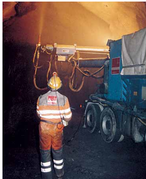
A shotcrete robot working its way through the Norwegian mountains.
