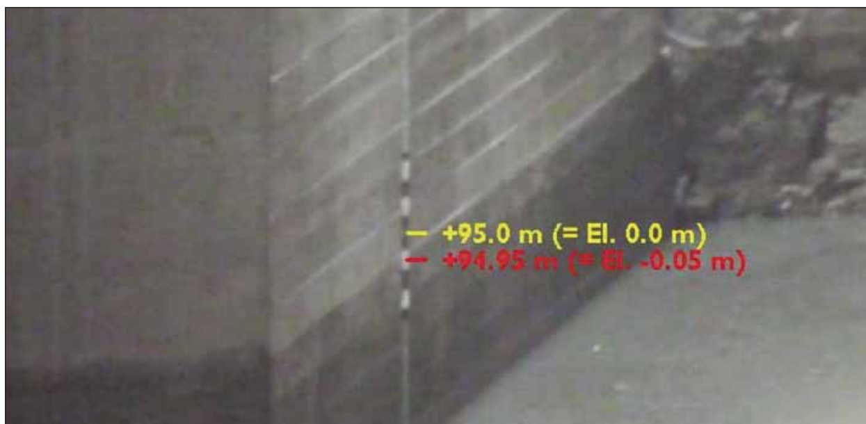
Figure 31: Maximum upsurge as wet markings on the stop log structure
