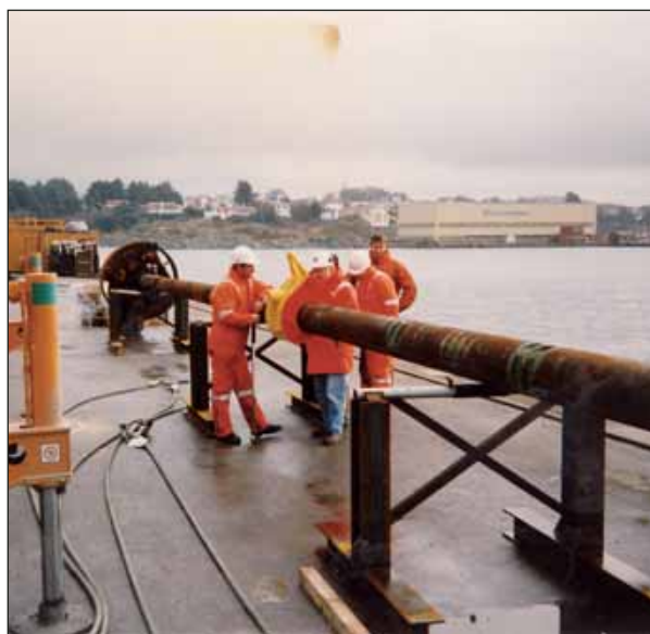
3. The reamer head connected to the drill string, prepared with lifting clamps and ready to be loaded onboard the supply vessel.
