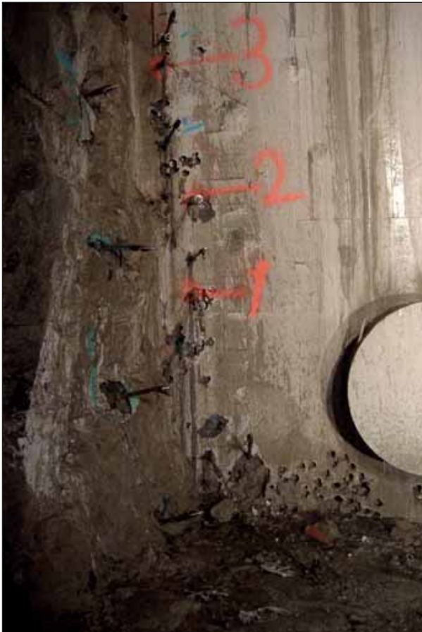
Re-grouting of Plug after too high leakages
