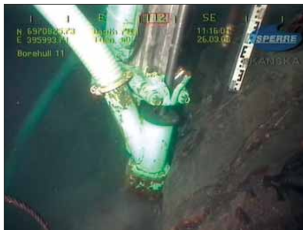
Figure 16 Drilling a blast hole
