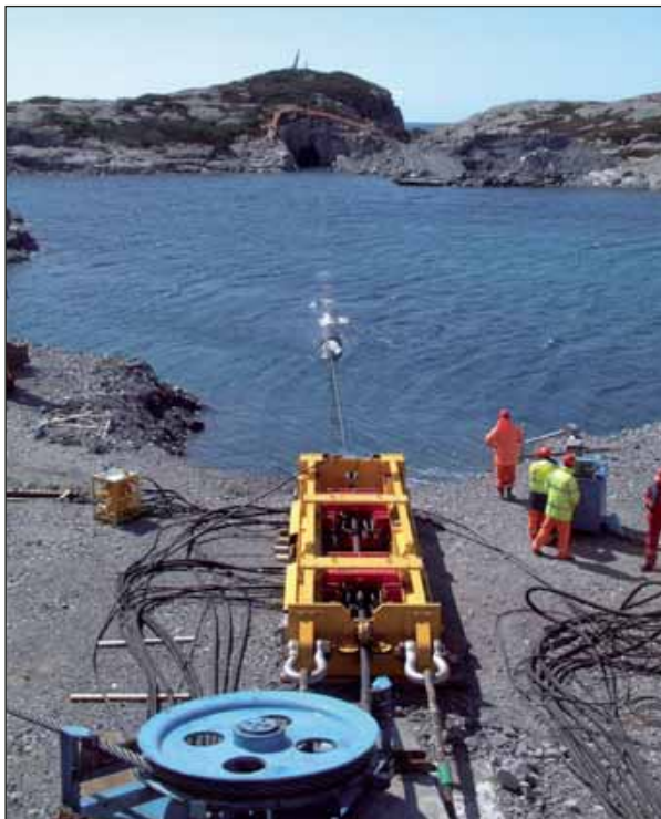
Figure 18: The pipeline being pulled over the strait. (Photo: Norconsult)
