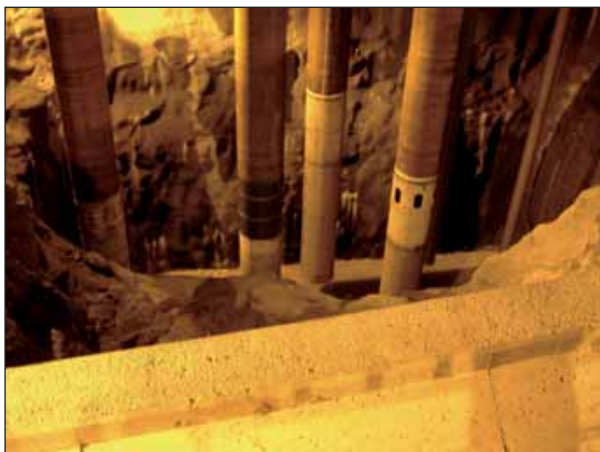
Sleeves in Pump Pit, Weir in front of Pit
