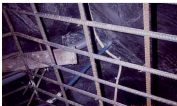
Pipes for cavity filling and air evacuation
