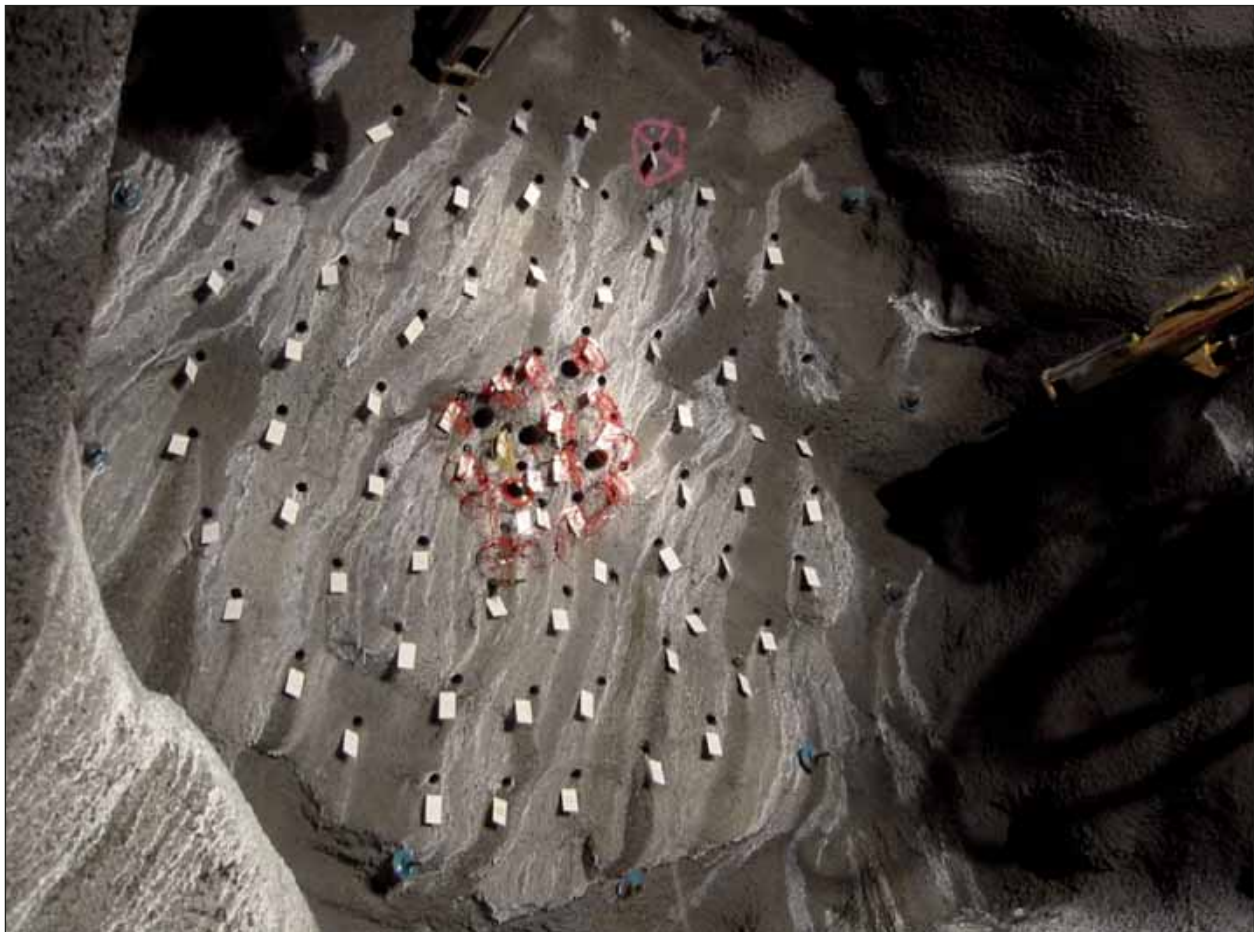
Figure 13: Drilling of underwater piercing blast round for Intake Tunnel completed. (Photo: AFS Pihl)
