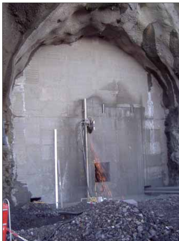
Re-opening of Access Tunnel
