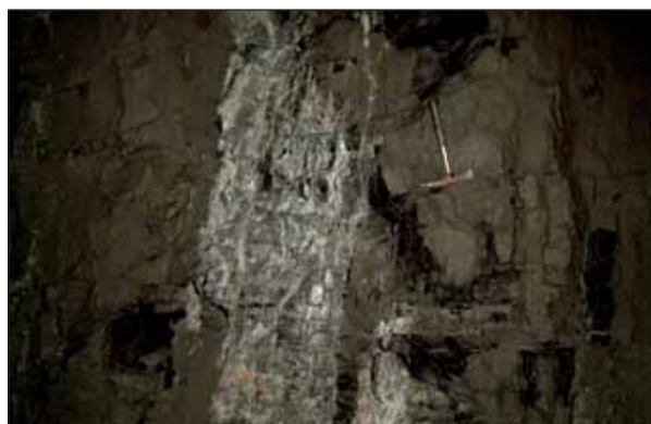
Figure 10: Tunnel portion with repeated parallel clay zones. (Photos: Statoil / Norconsult)
