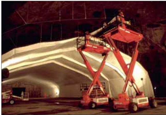
Installation of WG Tunnel Sealing System in rock cavern used for storage.
