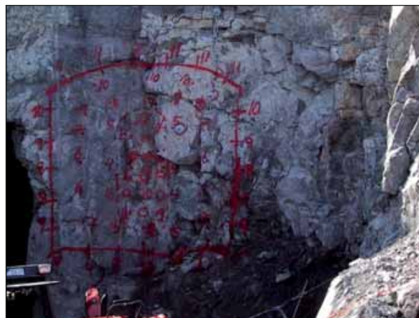
Figure 10: The actual ignition plan drawn on the entrance cut wall in scale 1:1. (Photo: Norconsult)
