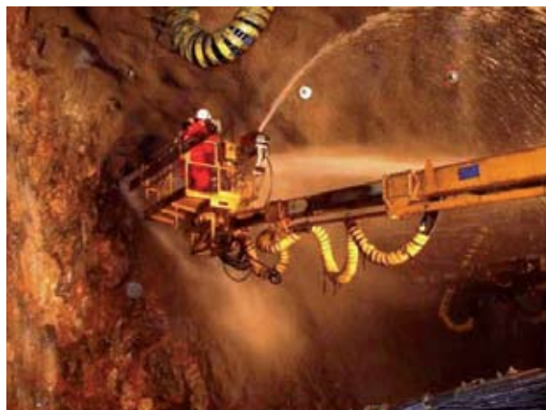
Figure 23. High pressure water inflow from probe holes (photo: CODAN/Ivar F. Andersen)
