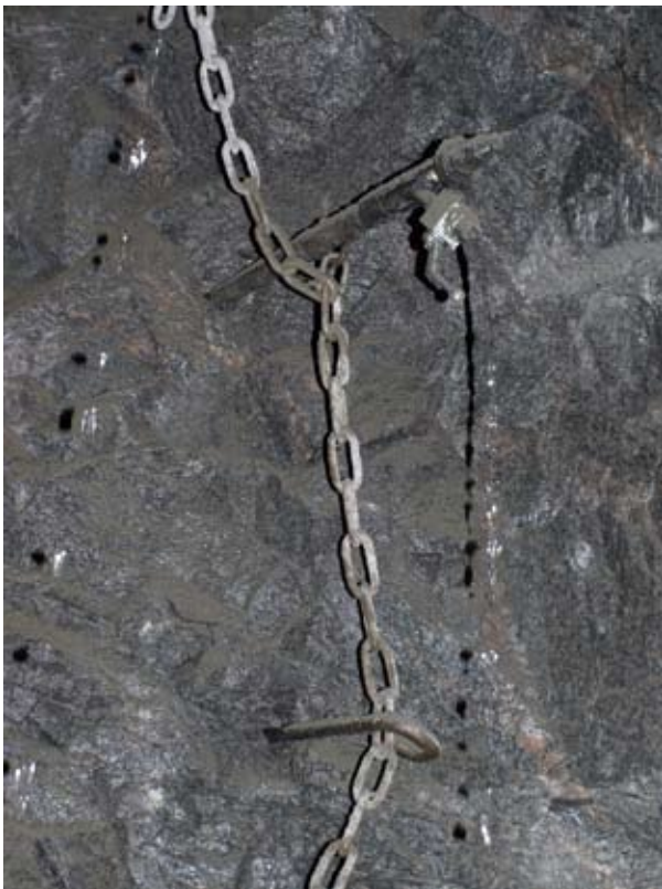
Figure 26. Grout packers secured by anchored chain. (Photo: AF Group/John I. Fagermo)
