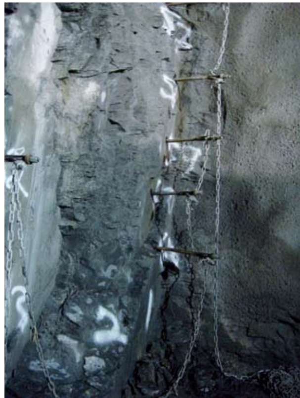
Figure 27. Grout packers secured by anchored chain. (Photo: AF Group/John I. Fagermo)
