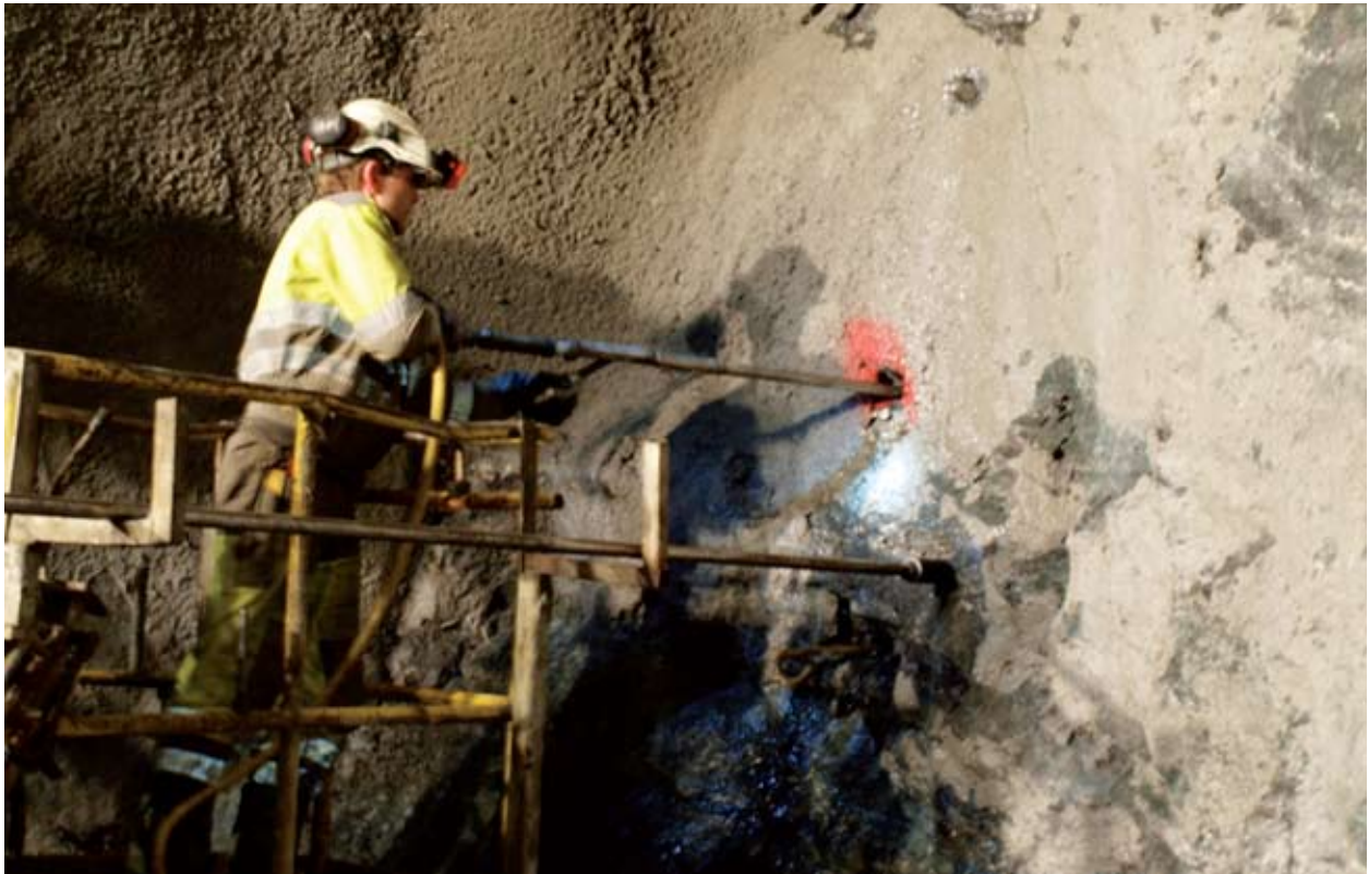
Figure 61. Insert and expand grout packer in grout hole (Photo: AF Group/John I. Fagermo)
