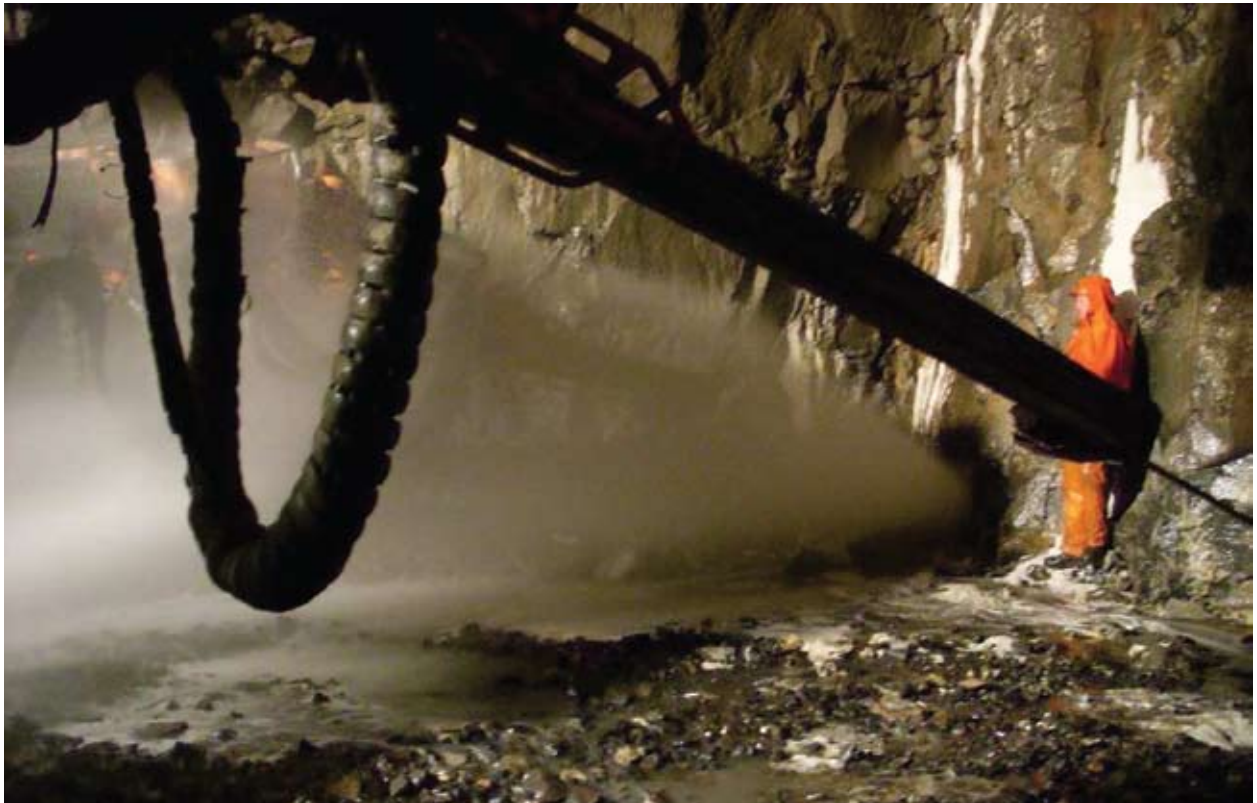
Figure 8. Example of a severe water inrush in a tunnel on Iceland (Photo: Bjørn Hardarson)
