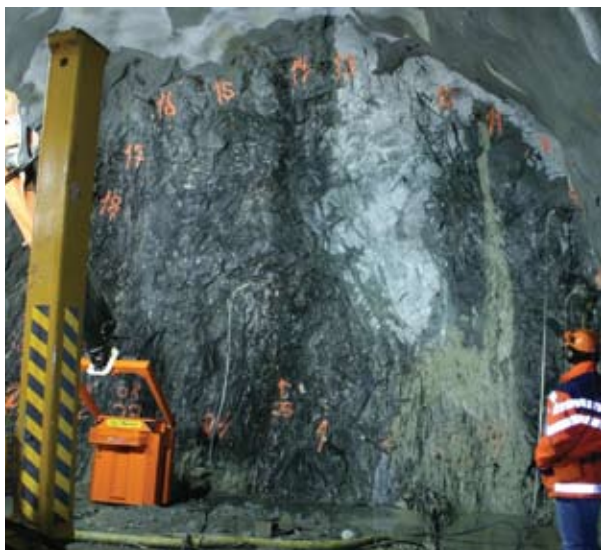
Figure 3. Preparing for grouting. Photo Svein Skeide, Statens vegvesen.
