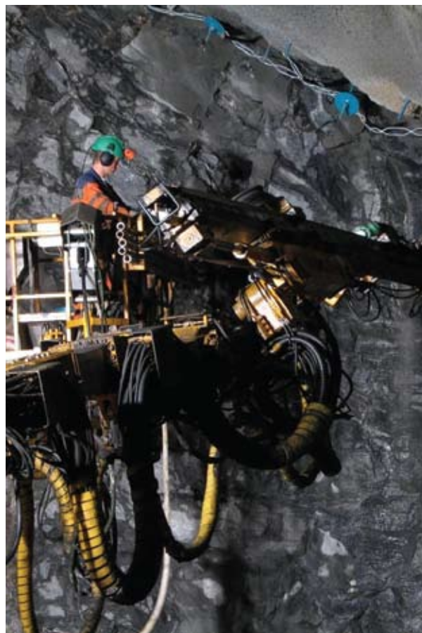
Figure 1. Investigation drilling at profile 1614, change of rod. Photo Svein Skeide, Statens vegvesen.
