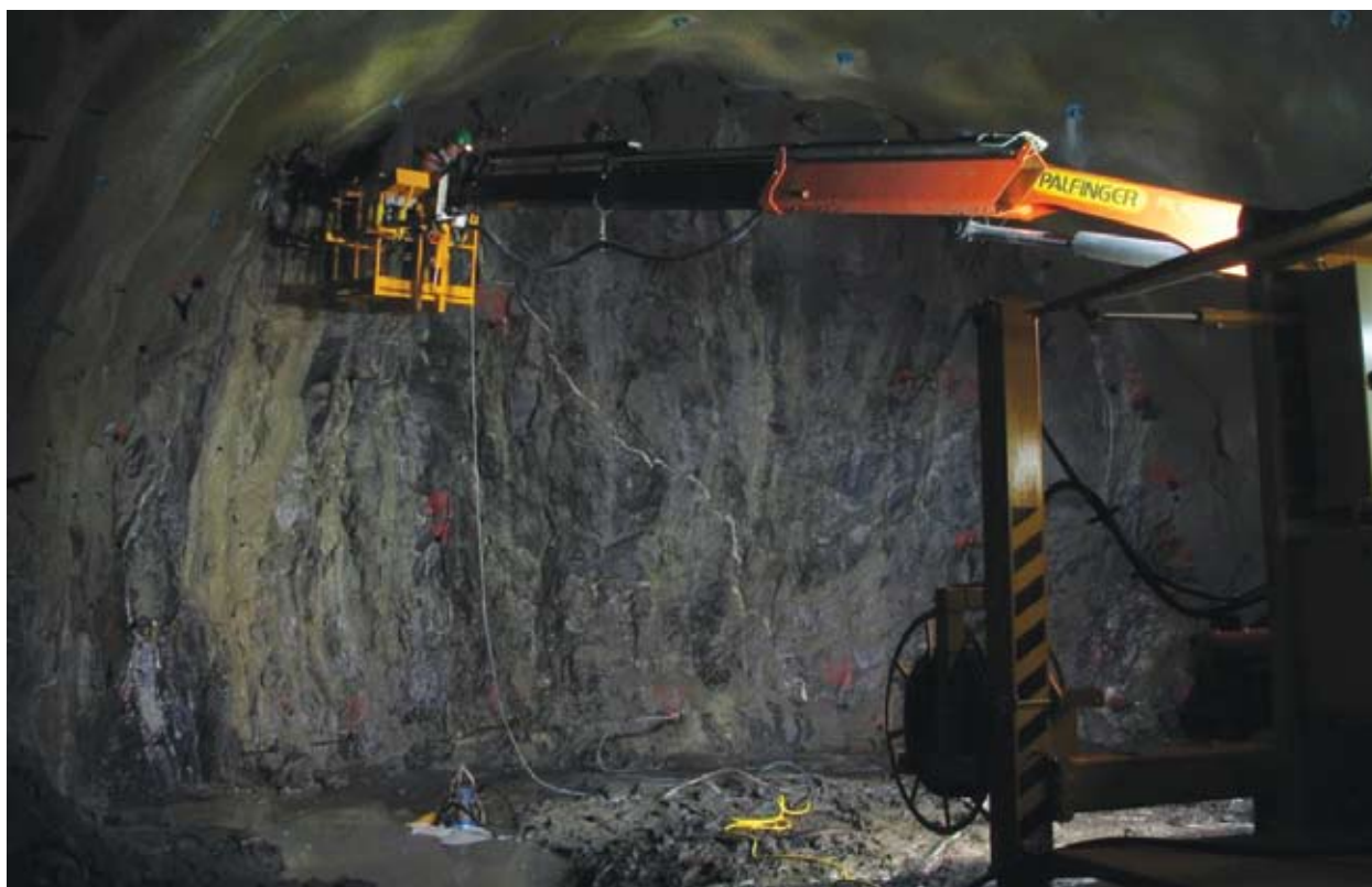
Figure 37. Injection in progress. Photo Svein Skeide, Statens vegvesen.
