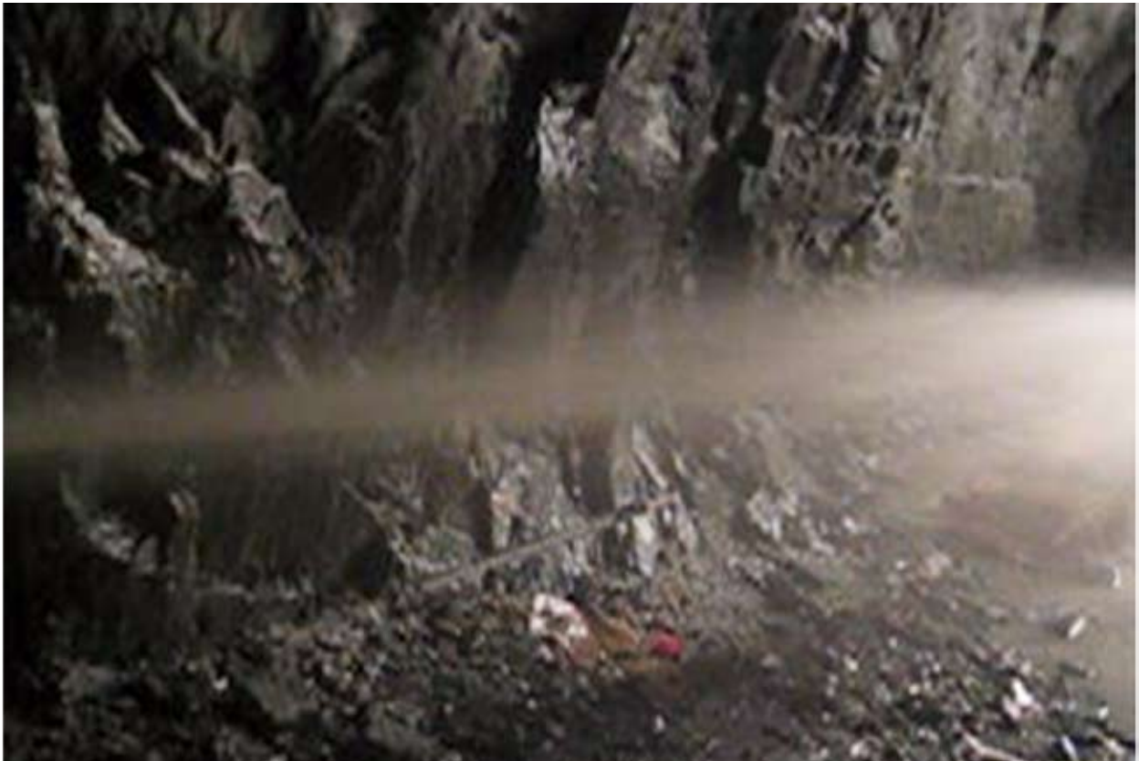
Figure 9. High pressure water inflow (Photo: AF Group/John I. Fagermo)
