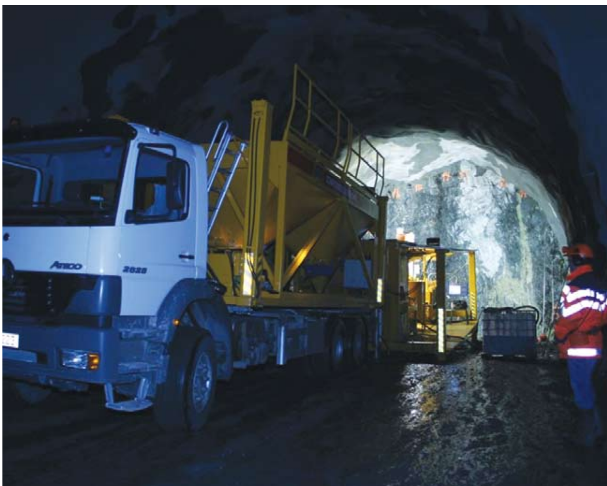
Figure 14. Modern grout rig in action (Photo Svein Skeide, Statens vegvesen.)
