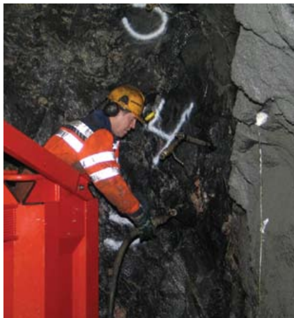
Figure 32. Operator moves packer. Photo Svein Skeide, Statens vegvesen.
