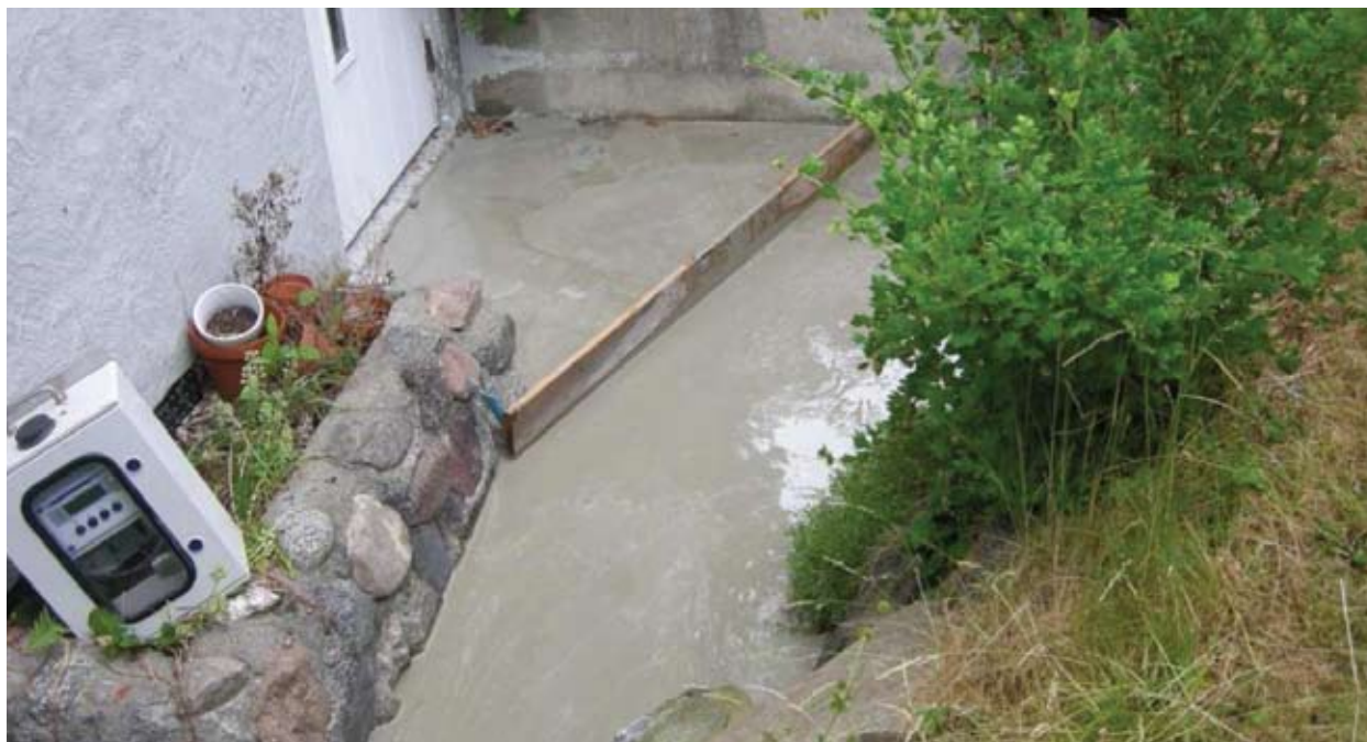
Figure 48. An example of migrating leaks at the surface
