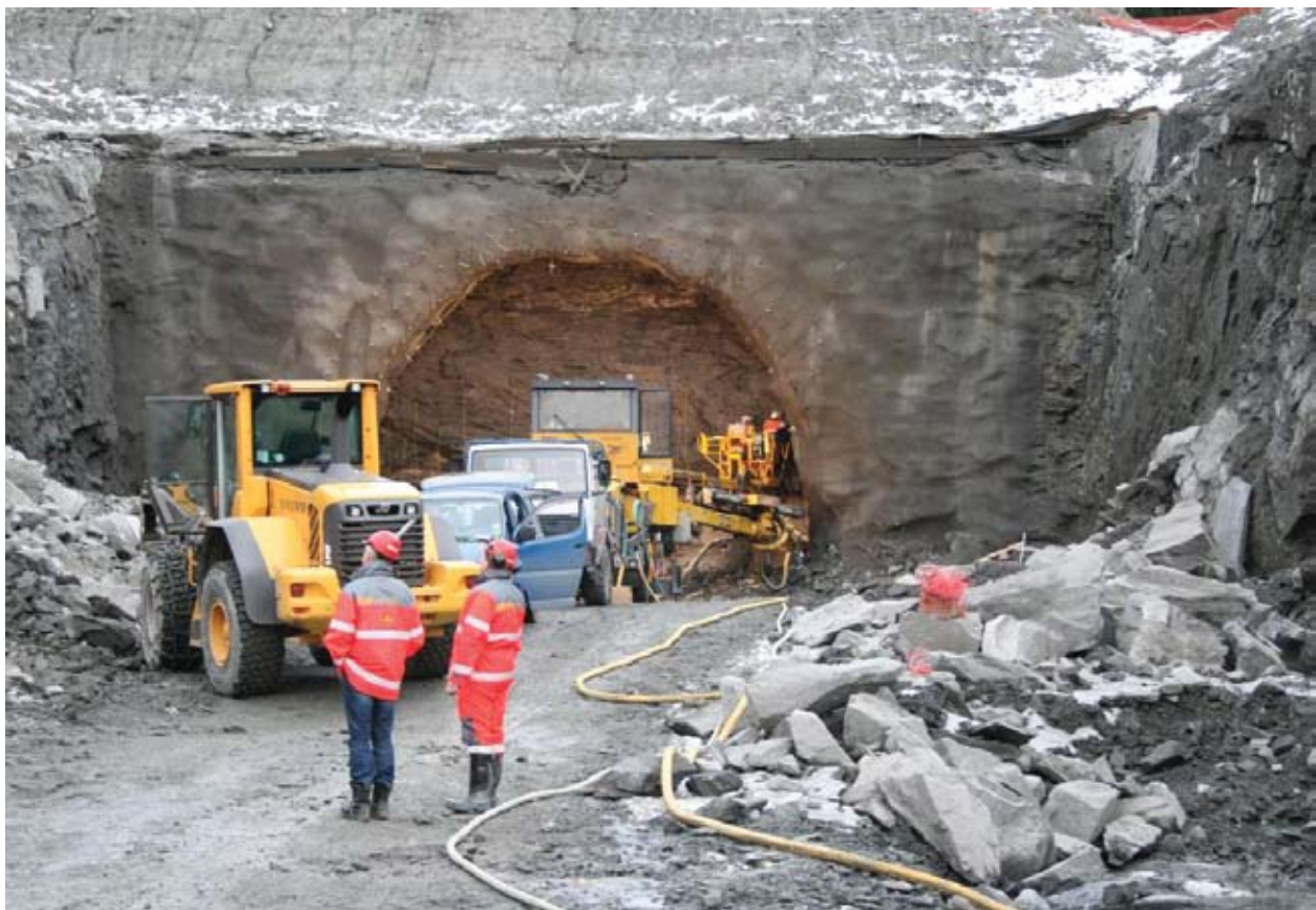
Figure 2. Tunnel cut for Eiksund subsea tunnel. Starting a descent of 300 metres. Photo Svein Skeide, Statens vegvesen.
