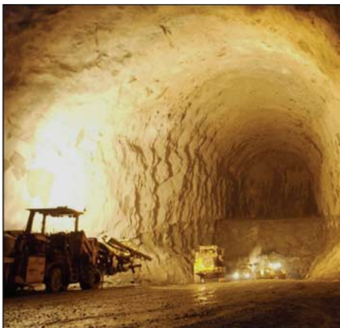
Figure 36. Excavation and grouting of the propane storage cavern at Mongstad.
