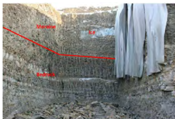
4b: Open cut excavation in moraine and weak rock (Photo Sverre Barlindhaug)
