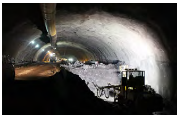
Figure 15: Excavation of the bench.
