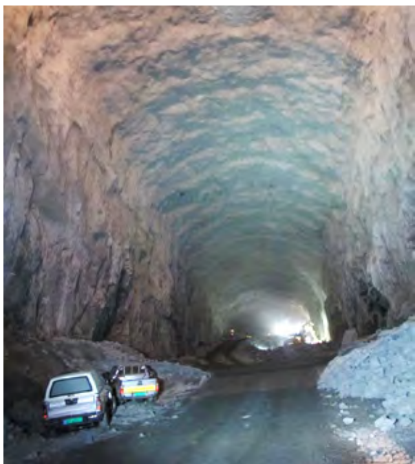
Figure 11. Fourth bench is starting in cavern 17.
