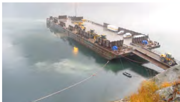
Figure 6: Barge used for controlled rock dumping into the 130 m deep fjord.
