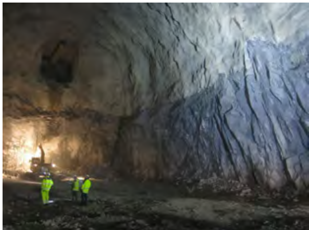
Figure 10: Scaling after excavating two benches in cavern 17
