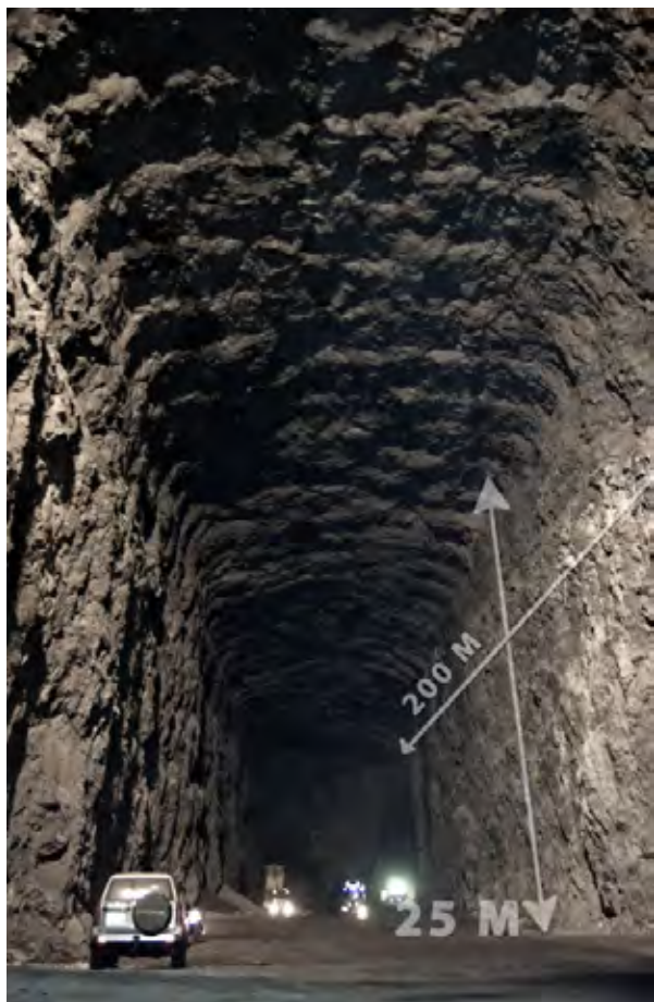
Photo 1: Rock cavern, 200 m long and 25 m high ( http://www.fsg.no/index.php/bilder/bilder-deponi )
