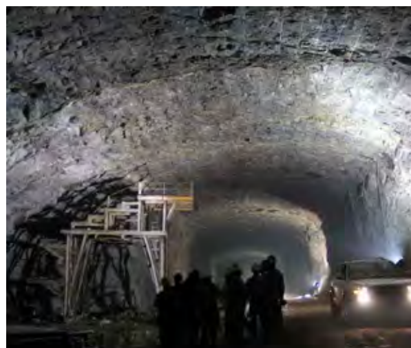
Figure 6 Excellent contour drilling and blasting in the 22.5m wide top heading showing very little overbreak
