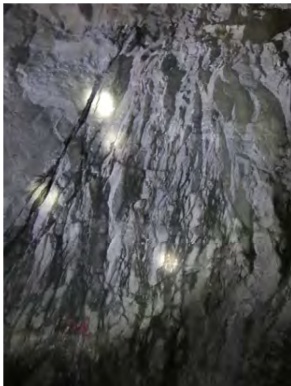
Figure 12: Typical stress- induced jointing patters in cavern no 18, necessitating use of shotcrete.
