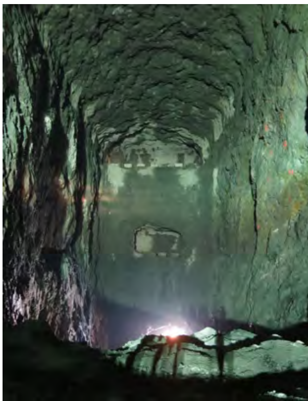
Photo 6. Photo showing access tunnels at different levels at the south end of the cavern. Photo by FSA, Multiconsult.
