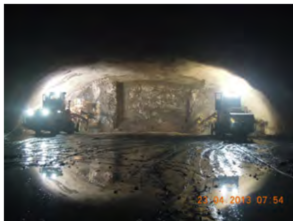
Figure 14: One round in the center of the gallery is excavated.
