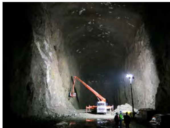
Photo 2: Lorry-mounted inspection platform for mapping and installation of rock support. Photo by FSA, Multiconsult.
