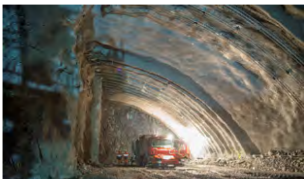
Figure 20. Lattice girder spacing c/c 1.0 m.
