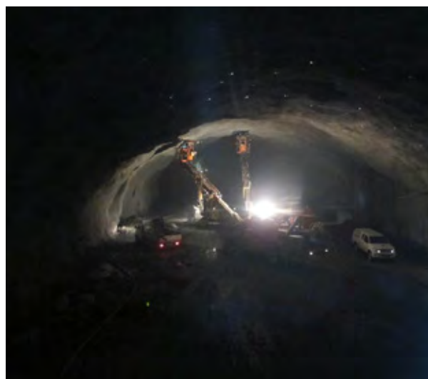
Figure 8: Installation of rock support in cavern 17.
