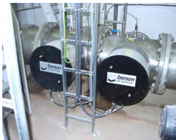
Figure 4: UV station temporarily installed in the old chlorine chamber
