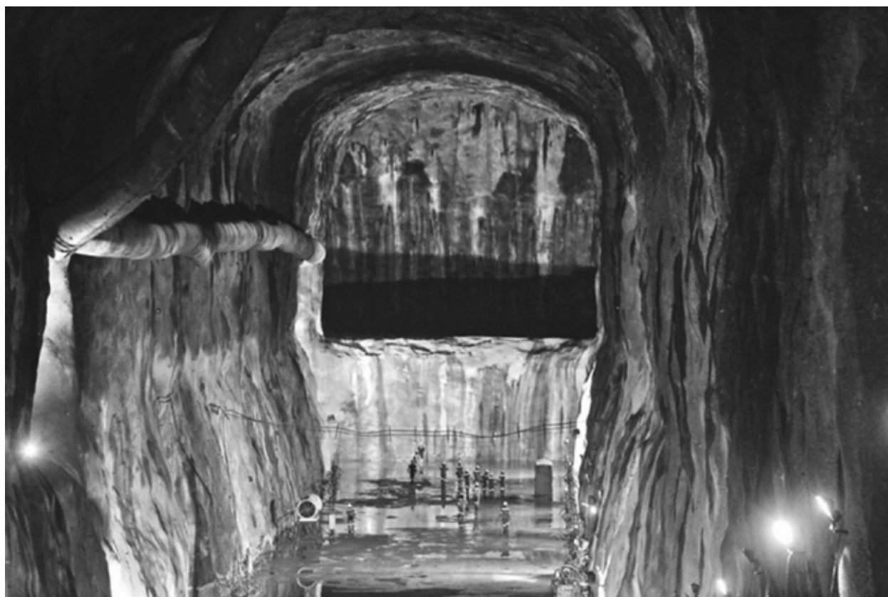
Figure 8: Rock cavern for hydrocarbon products, 165.000m 3
