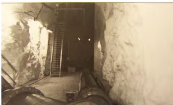
Figure 2: Pictures showing the entrance to the Steinan rock cavern tank and the inside with water pipe, concrete dam wall and shotcreted rock walls
