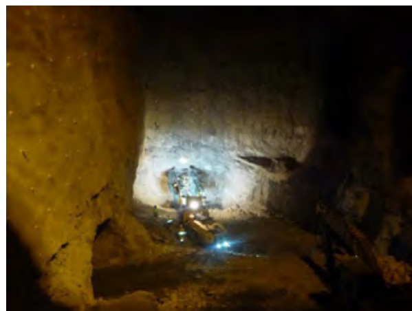
Figure 5. A: Ongoing drilling at the roof of main cavern (Stage 1). B: Excavating the cable tunnels. C: The crane is installed and the drilling has started again. D: Excavation of cooling water tunnel at the invert of the power station (Stage 3).
