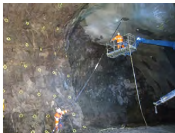
Figure 18: Installation of 12 m CT bolt.
