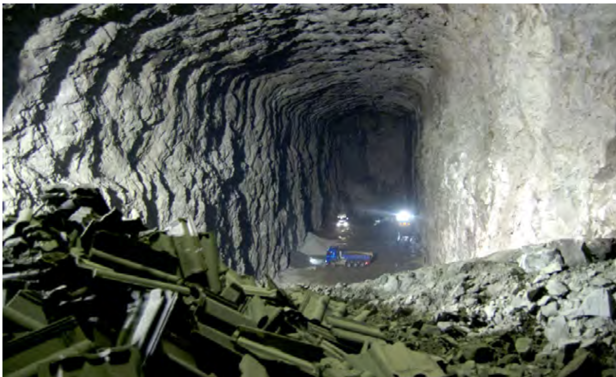
Photo 7. Inside the rock cavern, upper side, for waste disposal of contaminated masses. ( http://www.fsg.no/index.php/bilder/bilder-deponi )
