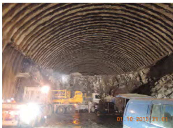
Figure 21. Excavation of the bench through the main fault zone.
