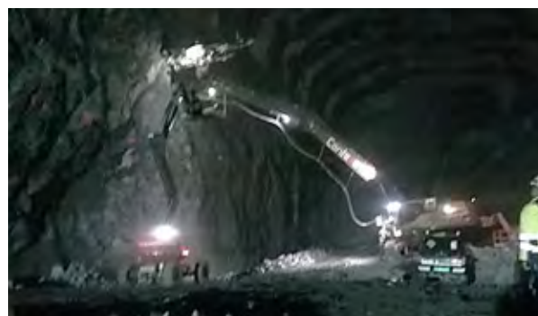
Photo 5: Installation of rock support in wall by drilling with long stick excavator with hydraulic hammer. Bolt installation is carried out by operator in a separate lifting platform. Photo by FSA, Multiconsult.
