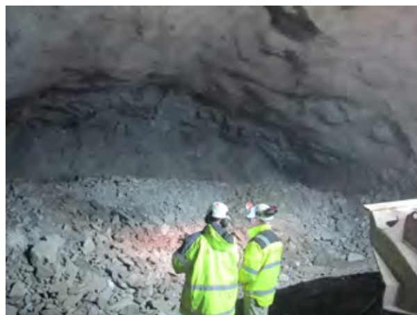
Figure 7: A completed blast of the top bench in cavern 17
