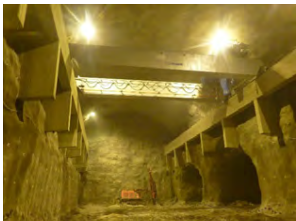
Figure 5. A: Ongoing drilling at the roof of main cavern (Stage 1). B: Excavating the cable tunnels. C: The crane is installed and the drilling has started again. D: Excavation of cooling water tunnel at the invert of the power station (Stage 3).
