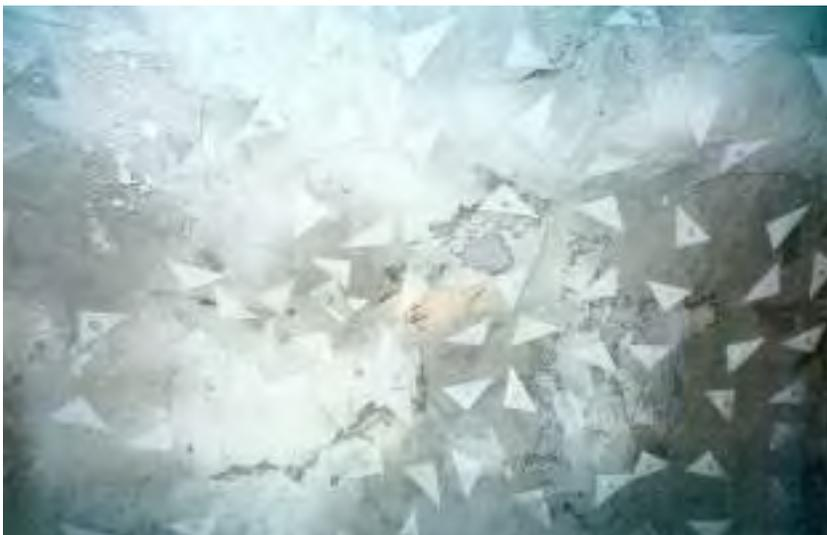
*Rock bolts equipped with triangular plates and net, in a tunnel subjected to rock burst.
