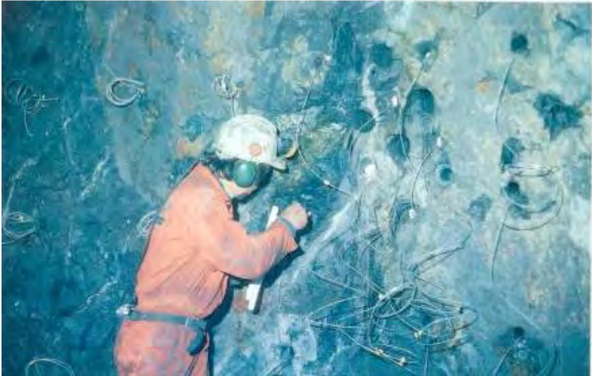
*The non-electric ignition system has many advantages and is coming more and more into use in tunnelling. (Norwegian Geotechnical Institute)*
