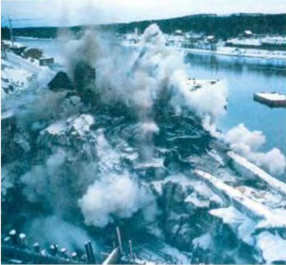
*Blasting of a massive rock cofferdam at Raanaasfoss power plant. The intake gates are located from 15 to 35 meters distance from the cofferdam (Norwegian Geotechnical Institute)*
