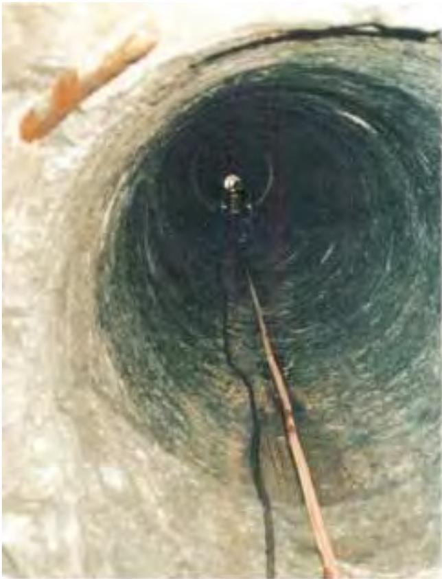
*Photo 16.3 A reamed shaft, diameter 1,5 meter (Entreprenørservice A/S)*
