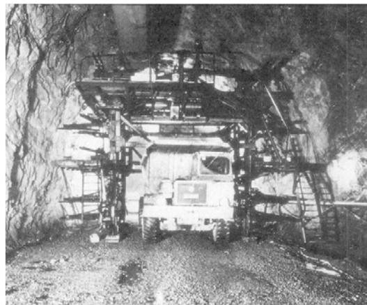
Fig. 1.5 Ladder drill rig at Nes power plant 1964
