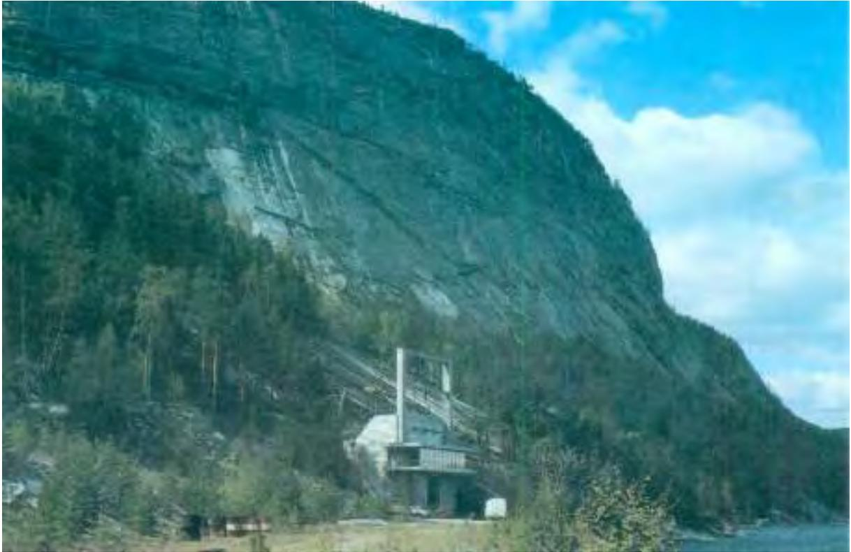
*The entrance of Fjone underground power station. This plant, subjected to high in situ rock stresses, had rock burst problems during construction. (Berdal)*
