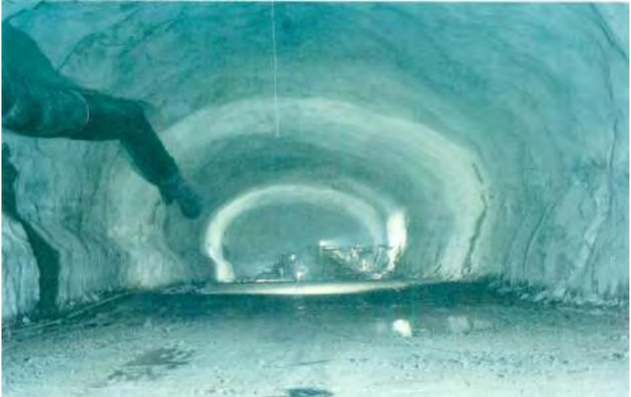
*The top heading of the Saurdal underground powerhouse. Roof support is carried out with fibercrete and systematic rock bolting. (Statskraft.)*
