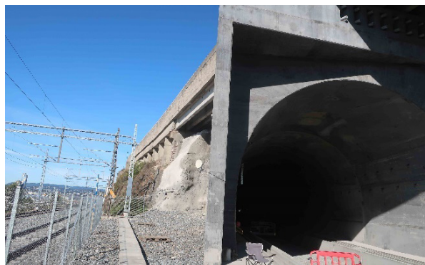
Figure 11-19: South Portal completed.
