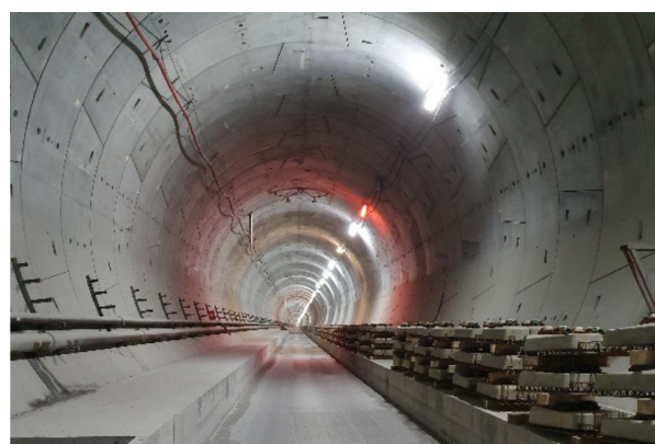
Figure 15-1: Segmental lining installed in the tunnel.
