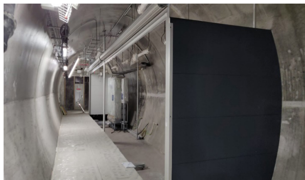
Figure 6-29: Cross passage safety egress.
