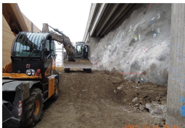
Figure 11-17: Rock support under the E18.
