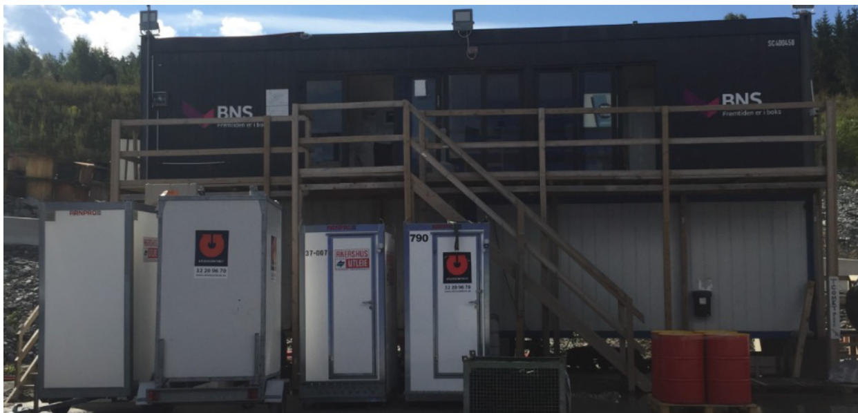
Figure 6-11: The Tunnel Control Center (TCC).
