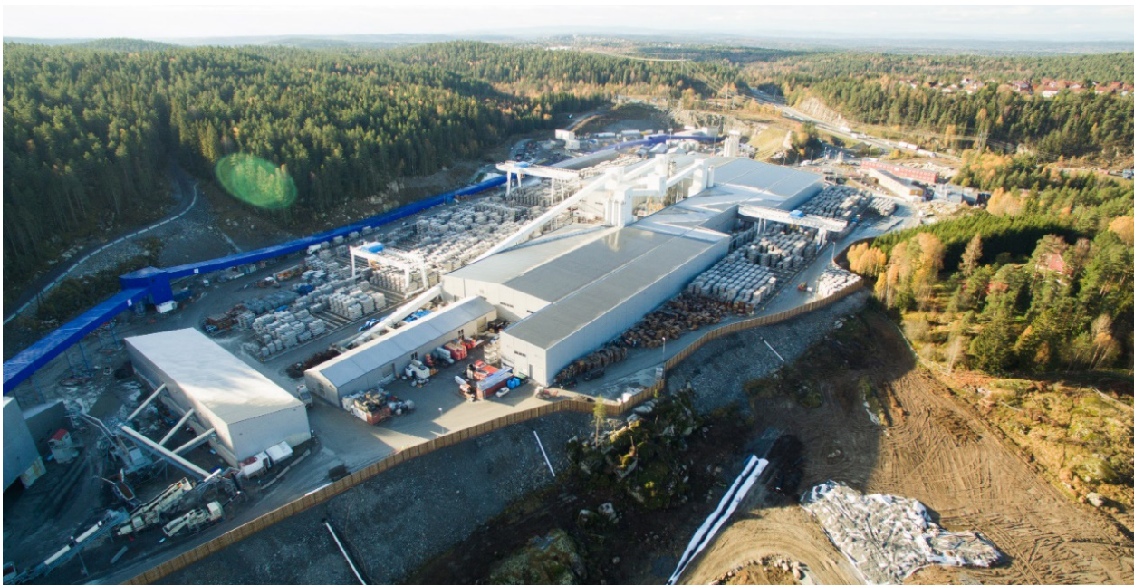
Figure 16-1: The spoil shed, crushing plant, aggregate shed, batching plant and the factories.
