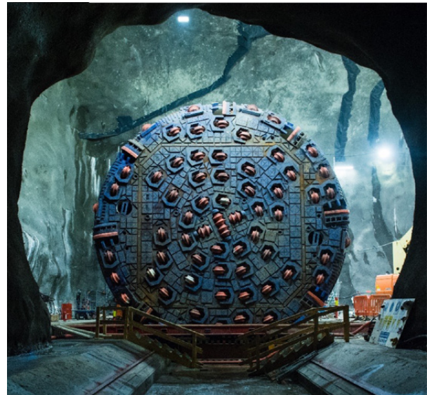
Figure 10-5: Launching of TBM S-982 (photo: Acciona-Ghella Joint Venture).
