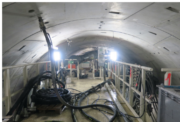
Figure 16-23: Secondary grouting through grout ports.
