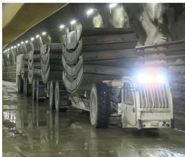
Figure 16-16: Transportation of the segments from the storage area to the TBMs.
