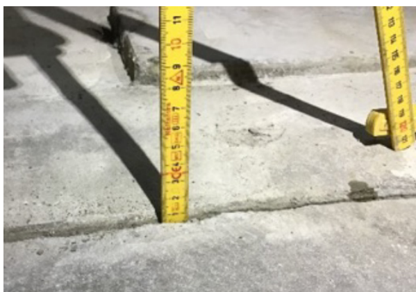
Figure 3: Left: Insufficient crack inducer. Right: Sufficient crack inducer.
