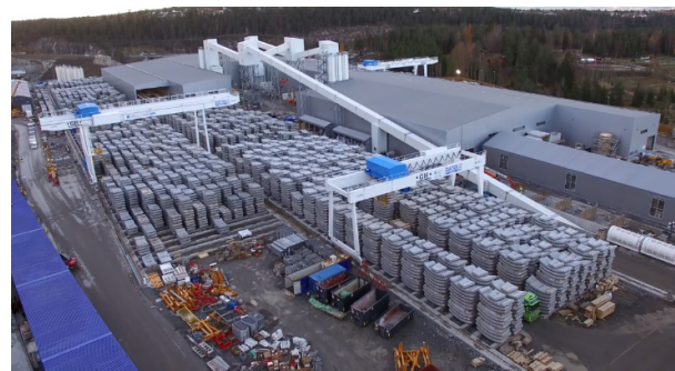
Figure 12-10: The three precast factories and segment storage area.
