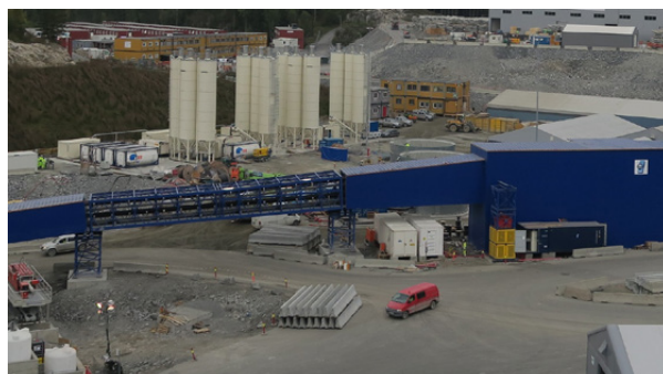
Figure 8-1: Sealed spoil conveyor under construction.
