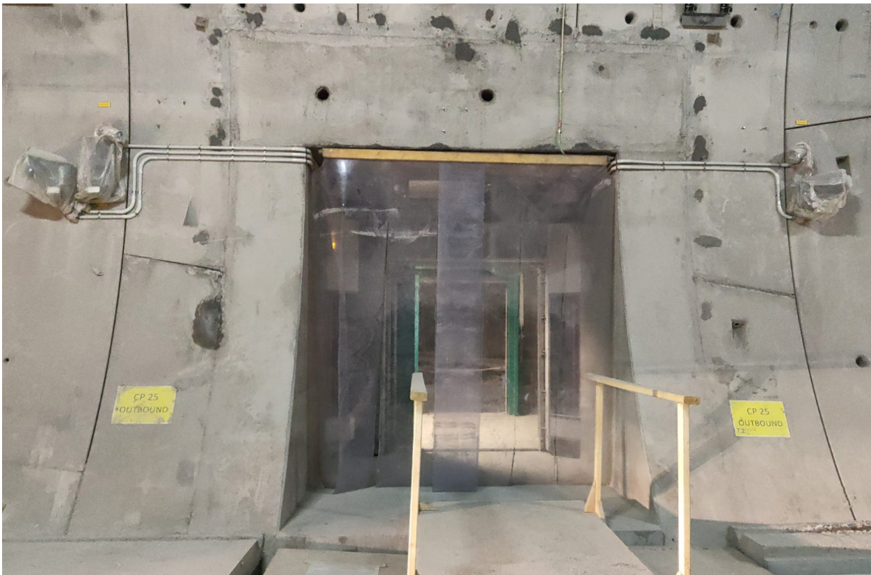
Figure 13-11: Open cross passage with temporary curtains during the construction phase.
