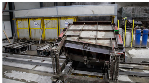
Figure 16-11: The carousel working line; Segment going into the curing chamber.
