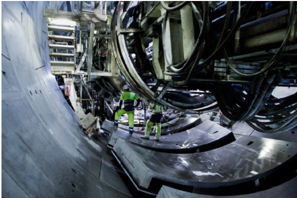
Figure 16-17: Feeding segments in the right sequence.
