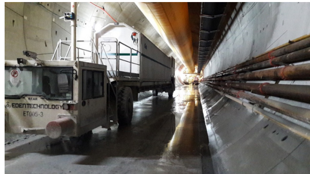
Figure 6-21: Rescue-vehicle with a refuge chamber.
