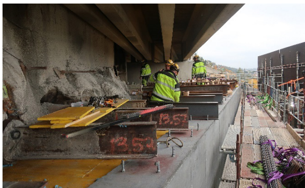
Figure 11-18: Extension of the H-beam.
