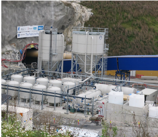
Figure 8-3: Water treatment plant under construction.
