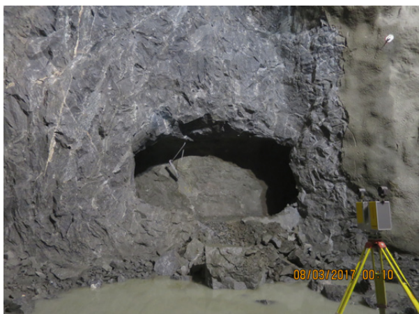
Figure 11-14: Careful blasting at the crossing.
