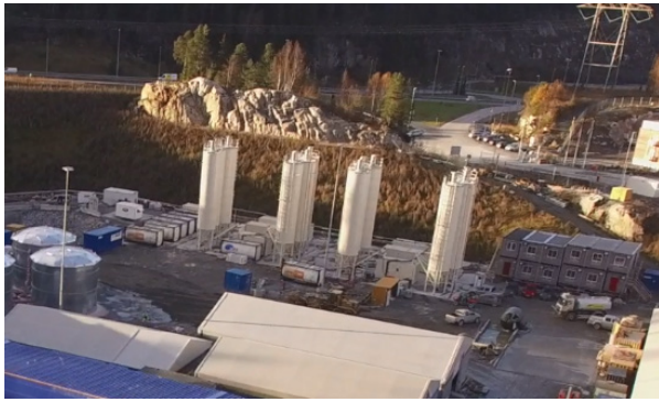
Figure 12-13: The grouting plant area.
