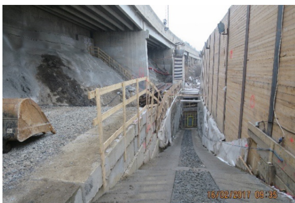
Figure 11-16: Access to the South Portal.
