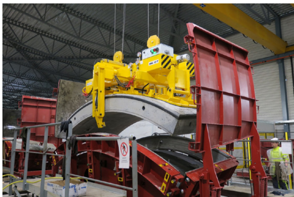
Figure 16-12: The carousel working line; De-molding station.
