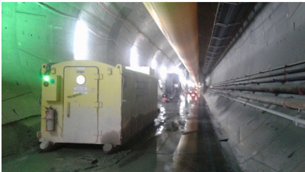
Figure 6-20: Refuge chamber for cross passages excavation.
