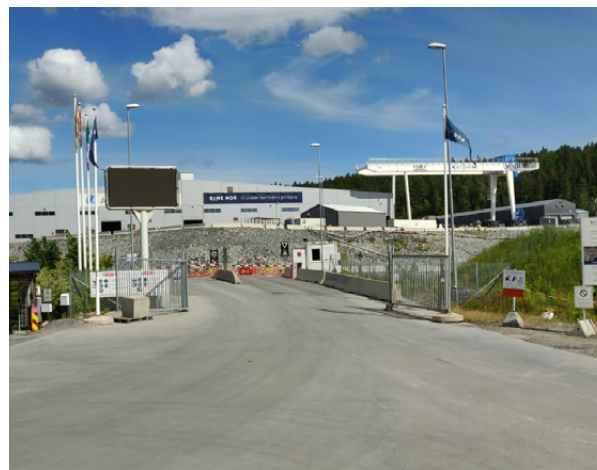
Figure 6-9: The main access to Åsland construction-site.
