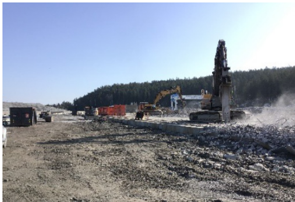
Figure 3.8.17. Hammering of concrete slab.
