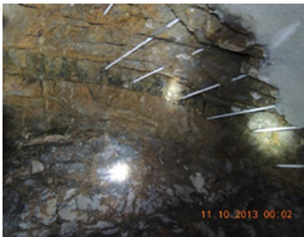
Figure 3.1.3. Left: Advance spiling bolts used to handle the zone described in figure 3.1.2. Right: RRS are installed on the face before continuing the blasting rounds.
