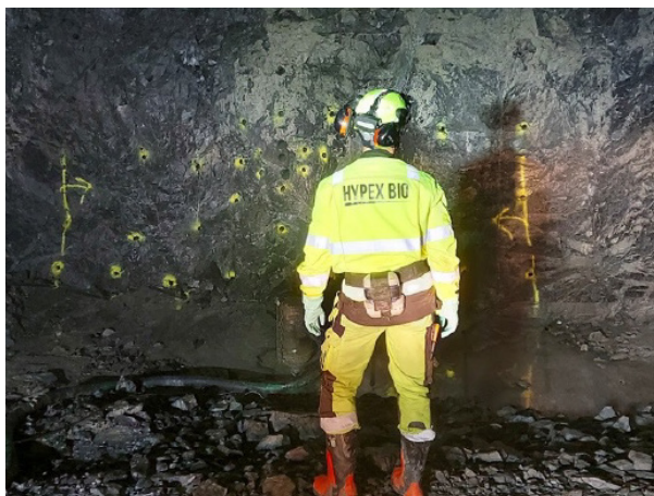
Figure 4.4.31. Pilot with Hypex Bio in a tunnel.
