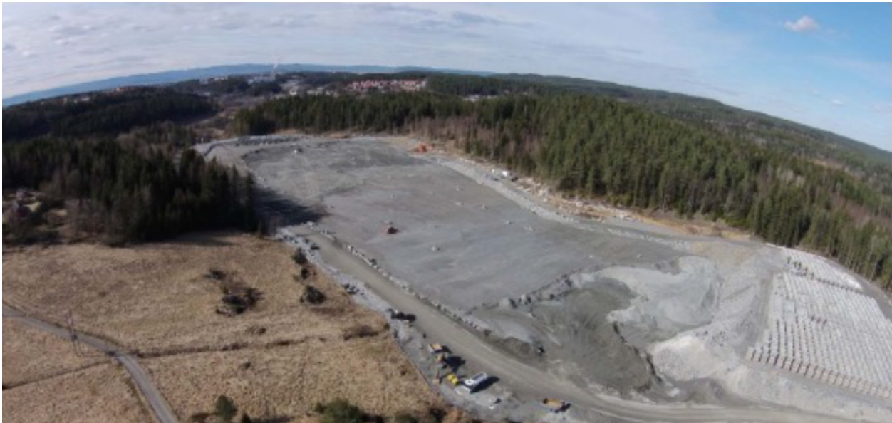
Figure 3.8.11. Overview of the TBM tunnel spoil deposit at the Follo Line, foundation of a future township outside Oslo (Photo: BaneNOR).
