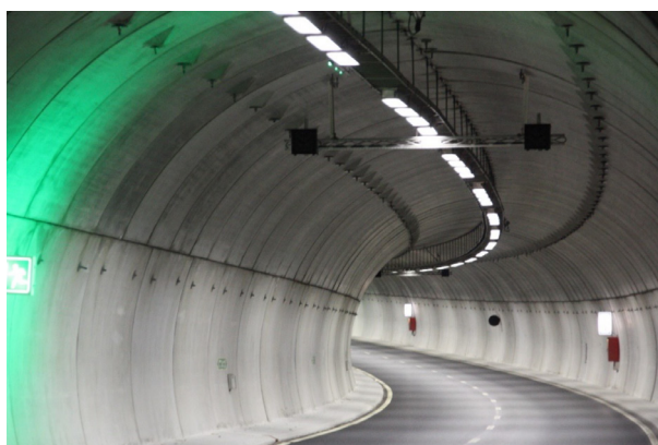
Figure 4.4.5. Concrete elements from Ølen.
