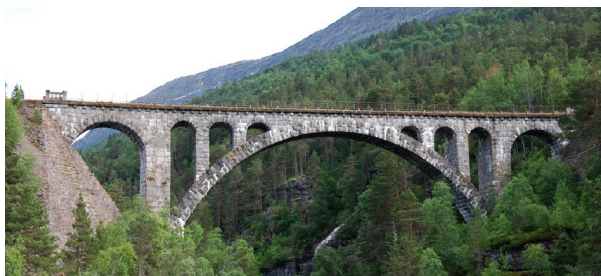
Figure 3.8.2. Raumabanan, the Arche Bridge made from masonry, natural stone.
