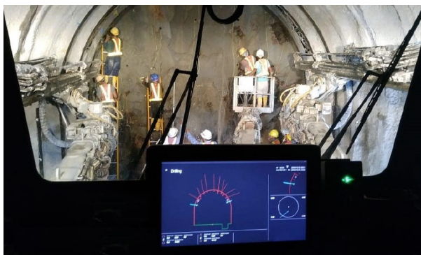
Figure 4.4.15. Drilling for a run-of-river hydropower plant in Sumatera, Indonesia. Photo: FMM.
