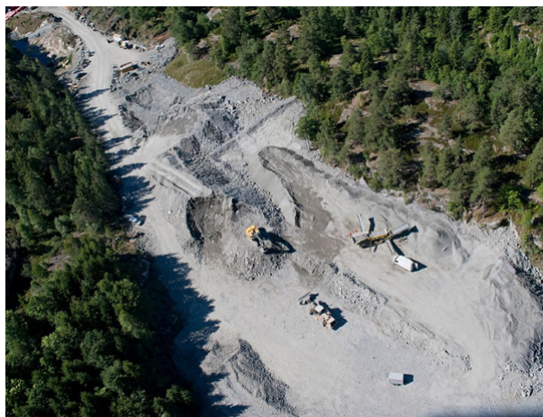
Figure 3.8.6. Crushing plant at the Vestfold Railway Project.
