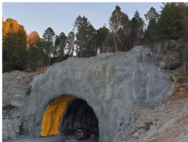
Figure 3.5.1. Burberg tunnel, aka. "The owl tunnel" in progress in November 2019.
