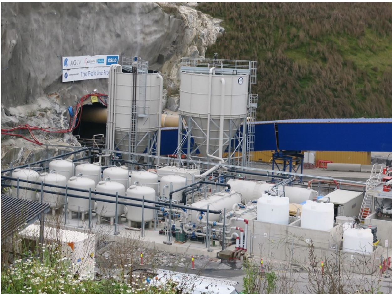
Figure 3.6.6. Water treatment plant under construction.
