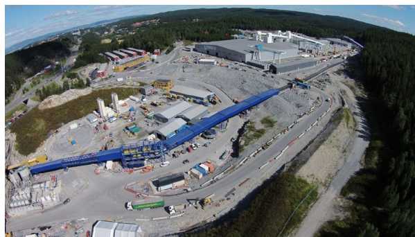
Figure 3.8.9. An overview of the Follo Line construction plant at Åsland.
