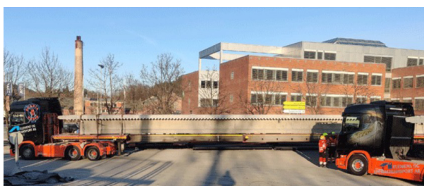
Figure 4.3.11. Heavy duty: The bridge is carefully transported to Nesbyen. Photo: IMIS ( https://nyheter.byggfakta.no/ta-en-bru-og-la-den-vandre-196490/nyhet.html ).
