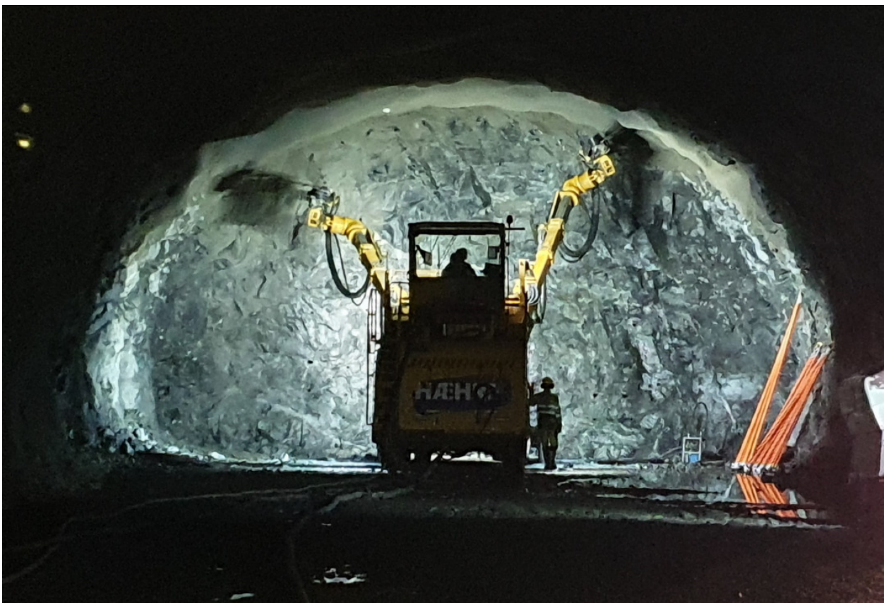
Figure 4.3.5. Tunnelling on the E16 Kvamskleiva project (Photo: Tommy Hagen, Hæhre).
