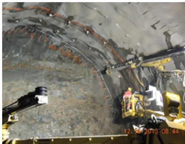
Figure 3.1.3. Left: Advance spiling bolts used to handle the zone described in figure 3.1.2. Right: RRS are installed on the face before continuing the blasting rounds.
