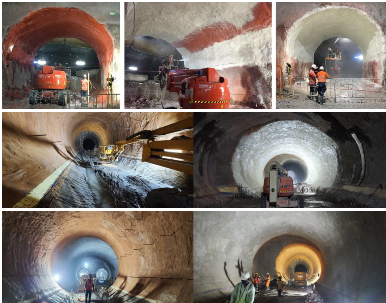
Figure 4.4.11. Examples of shotcrete surfaces.
