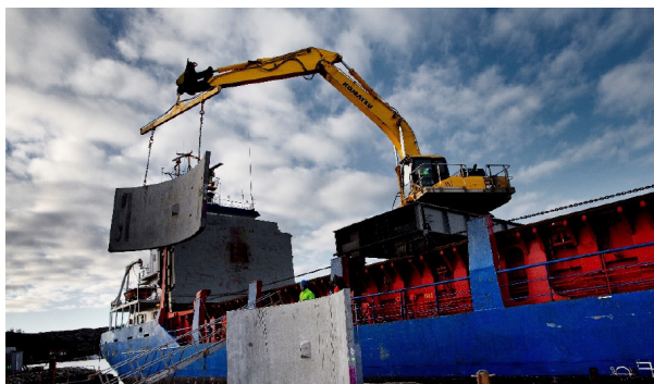
Figure 4.4.7. 2 Loading tunnel element quayside in Mølstrevåg.
