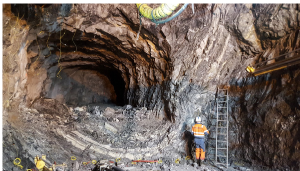
Figure 3.8.9. Charging a new round at the OREA sewer project in Strømmen near Oslo (photo E. Hannestad, Sweco Norge AS).
