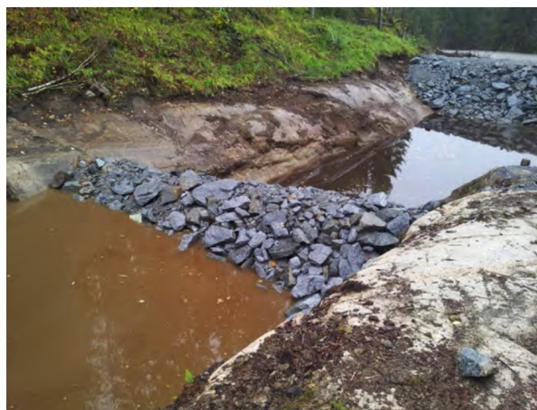
Figure 3.6.5. Sedimentary basins as a simple process to clean draining water from deposits of tunnel muck.
