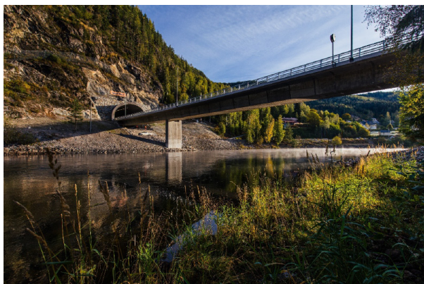
Figure 4.3.2. Bagn - Bjørgo, the bridge leading directly into the tunnel (Photo: Skanska).
