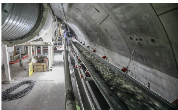
Figure 3.2.4. 9 million tons of spoil transported on conveyor belts.
