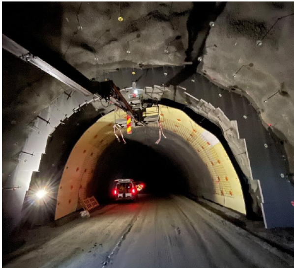
Figure 4.4.3. Foamrox used as fire barrier between tunnel sections.
