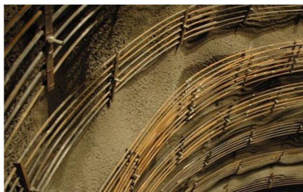
Figure 3.1.3. Left: Advance spiling bolts used to handle the zone described in figure 3.1.2. Right: RRS are installed on the face before continuing the blasting rounds.
