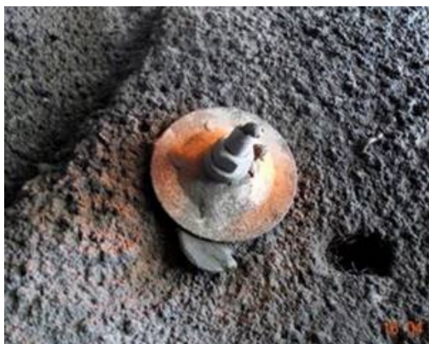
Figure 4.12 Complete filling of hole and combination bolt. Photo Terje Kirkeby
